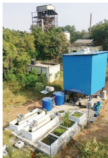
Fig. 13: Waste Biorefinery: Integration of multiple bioprocesses (anaerobic digestion, algal cultivation, anoxic system, bioelectrogenic system, Ecologically Engineered system) with biohydrogen production for multi-product recovery
