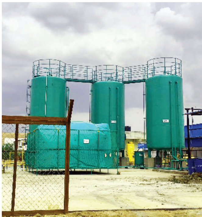
5 TPD biomethanation plant based on AGR at Jawahar Nagar, Hyderabad
