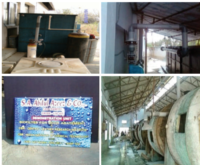
Full scale Bio-filter for odour removal in Tannery
