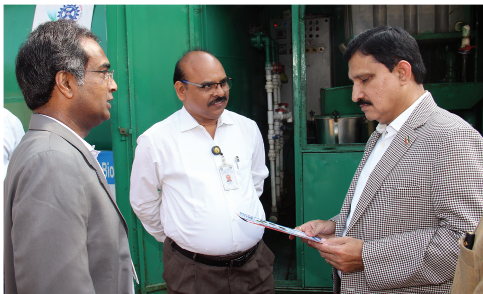
Senior Scientist Dr. A. G. Rao and Director, Dr. S. Chandrasekhar explaining the installation and functioning of Anaerobic Gas Reactor
